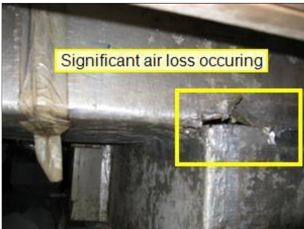
6.3 Picture 4 crawlspace new addition
