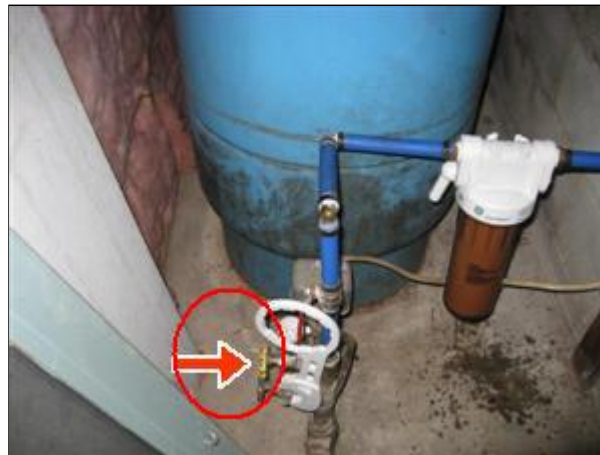
4.3 Picture 1 In basement
