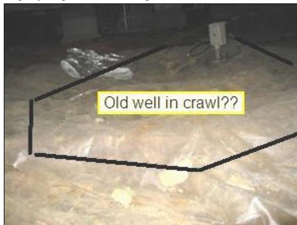
2.6 Picture 2 in crawlspace under new addition
