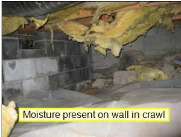
1.0 Picture 5 crawlspace under kitchen
